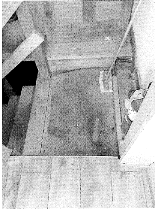
Water-damaged carpet on cellar stair threshold
