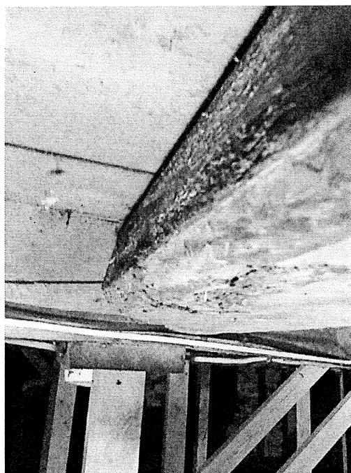
Mold colonization on surface of floor beams
