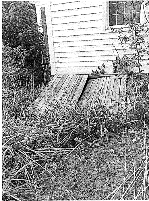
Damaged bulkhead doors
