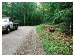
Mud-season rutting: Rutting that developed during the mud season required emergency repairs. Stone used to help make the
