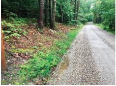
• Standing Water: Standing water at the edge of roadway highlights the importance of proper ditch maintenance and design. This is especially important before the winter/spring months when the freezing and thawing of trapped water can cause roadway heaving. Some areas with slate have made the recommended 2'-3' depths difficult to achieve.
