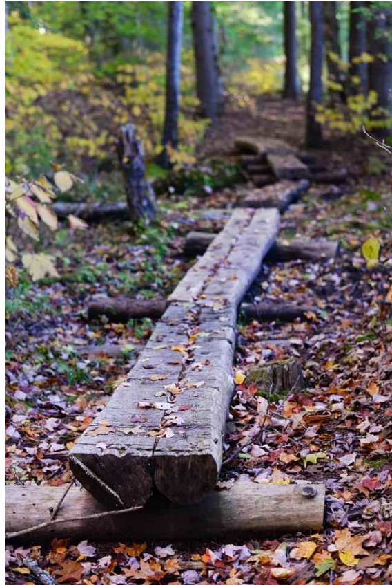
Bog bridge at Pelham Lake Park
