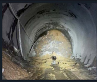
TOP: site of the cave-in BELOW: Cave-in from inside the tunnel.
