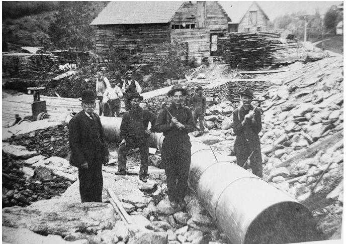
Water power conduit for the talc mill.
