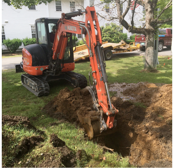
Lynde Well Drilling trying to locate leaking pipes
