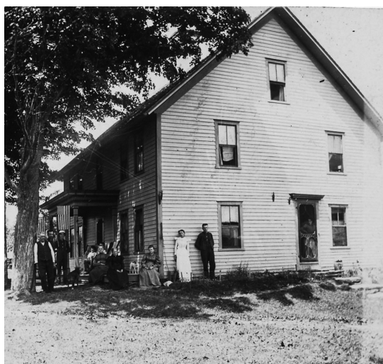
There was the "Maple House" at 51 Middletown Hill Rd. (Bradley) with boarders first noted in 1887. The Bradleys continue to hosts guest there year round.
