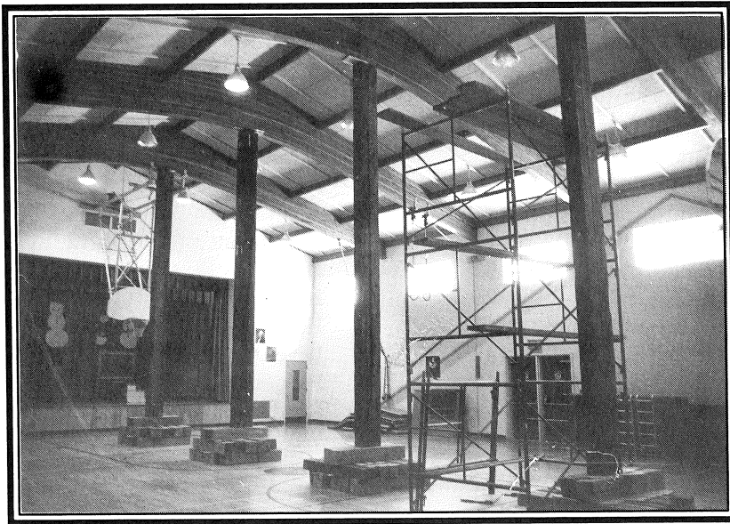
Massive supports hold cracking roof trusses at Rowe Elementary School.
